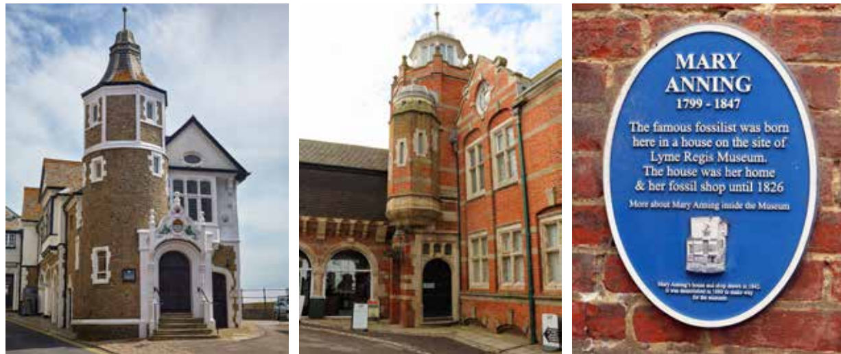
Left to right: The distinctive Italianate Guildhall, with its rounded tower, on the corner of Church Street and Bridge Street, offering views to the sea; equally impressive Lyme Regis Museum and lantern tower, with its rich stone; a blue plaque commemorating fossil hunter Mary Anning, who is celebrated at the museum.
